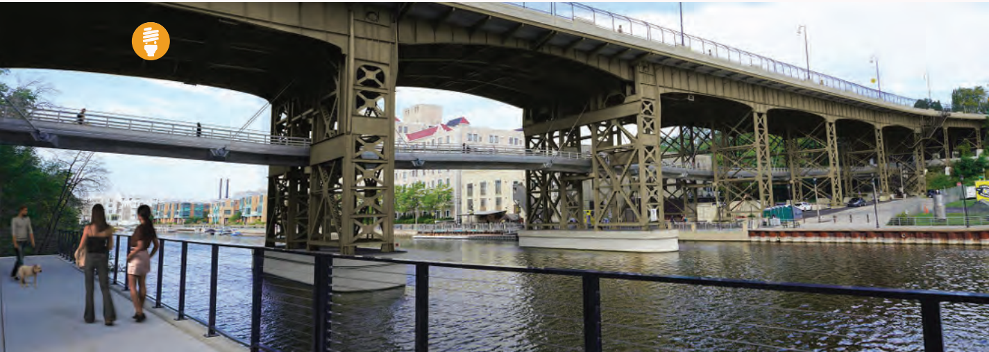
Holton Viaduct Marsupial Bridge The Holton Street Viaduct Marsupial Bridge (2004-05) transformed unused space beneath an existing viaduct into a pedestrian/bike path linking Milwaukee neighborhoods. Similar infrastructure beneath I-90 and I-391 could link Holyoke to the Connecticut River Bikeway.
